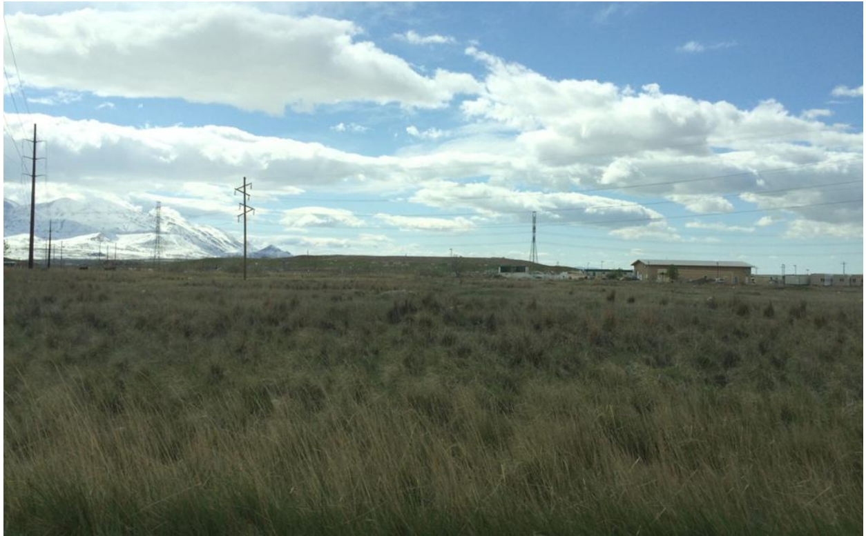
View west toward the landfill from 5600 West. The east edge of the landfill can be seen on the horizon. The landfill currently rises to approximately 75 feet in height.
