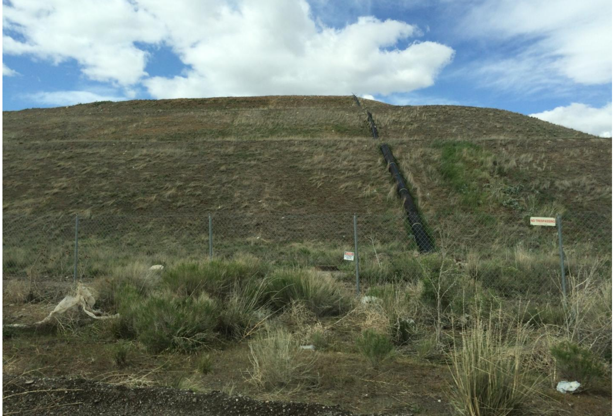
Close up view looking north from California Ave showing existing 150' tall landfill
